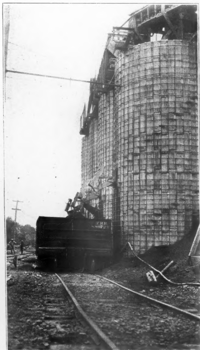
Freight Cars Loading at Concrete Stave Bins
